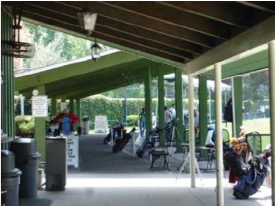
N: Driving Range Shelter (ARG)
