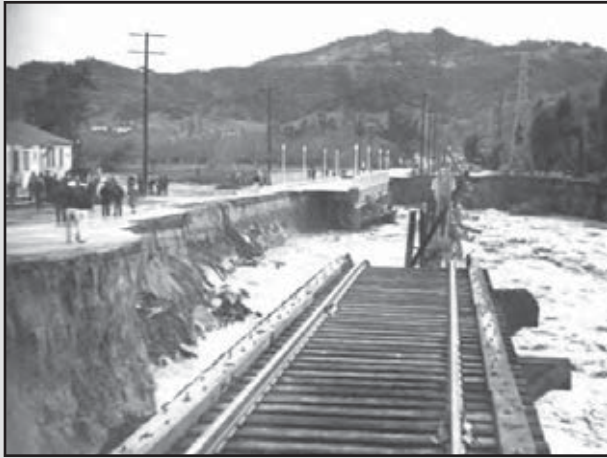
L.A. River Flood Damage, Vineland Ave., 1938 (CSUN Library)
