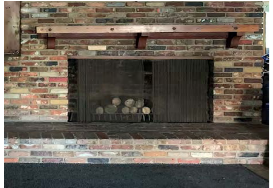
D: Clubhouse Interior: Fireplace (June 2020)
